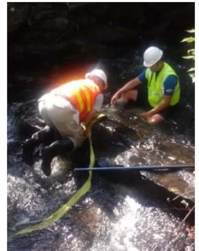
The team discovered—and successfully removed—several blocks that were affixed to the bottom and caused an abrupt break in the channel profile.
